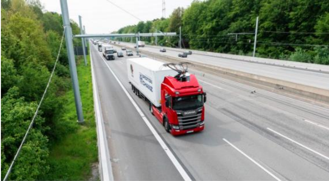
Figure 9 – Electrified road system trial 45
